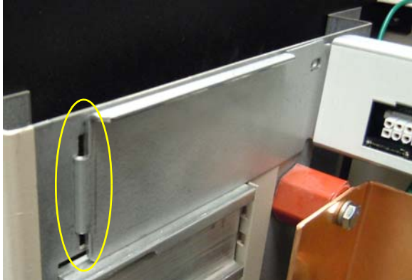
Slide arm clips in place to ensure proper screw alignment
